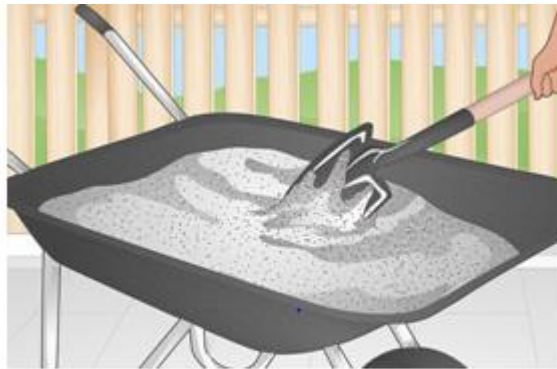
Fig: 3.3 Mix the dry ingredients
