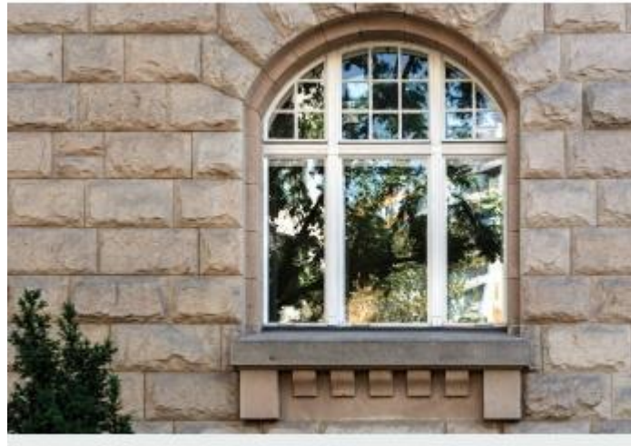
Fig3.4 stone cladding
