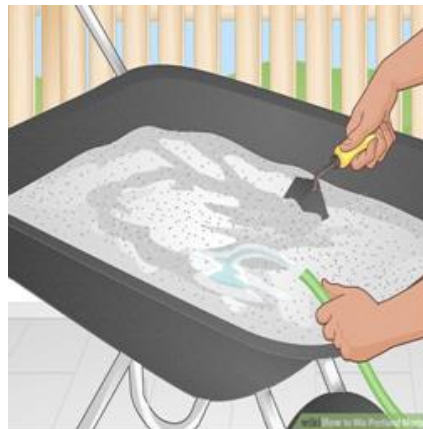
Fig: 3.3 Add water to the dry ingredients
