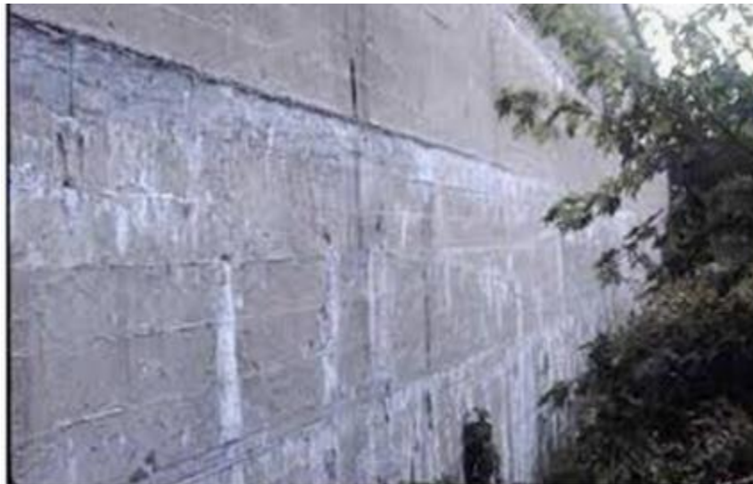
Fig: 4.1. Efflorescence on a concrete wall.
