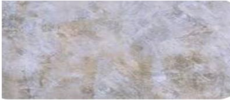
Fig: 4.1. Discoloration of concrete wall
